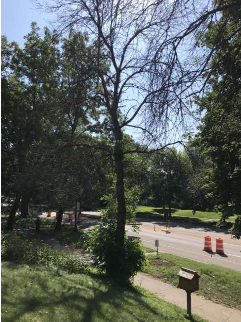
2163 Marshall Ave. Photos 8-23-23
